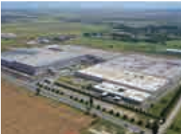
ROMANIA Romania Plant
