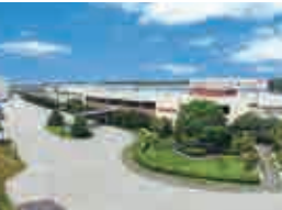
CHINA China Plant (MCC)
